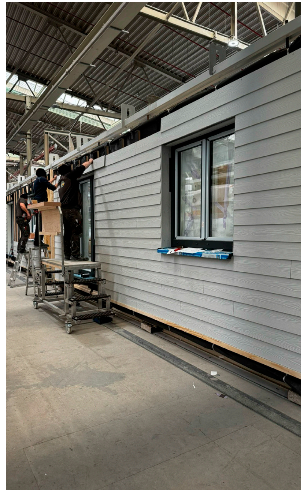
Façade element for serial renovation in prefabrication
